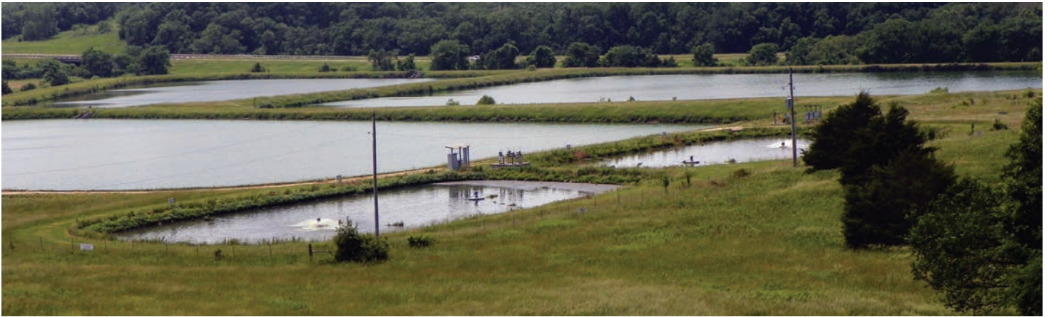
The current south sewer lagoons will be replaced with a wastewater treatment facility that should be sufficient for Louisburg's needs for the next 20 years.
